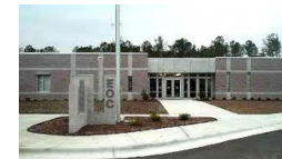
Emergency Operations Center
